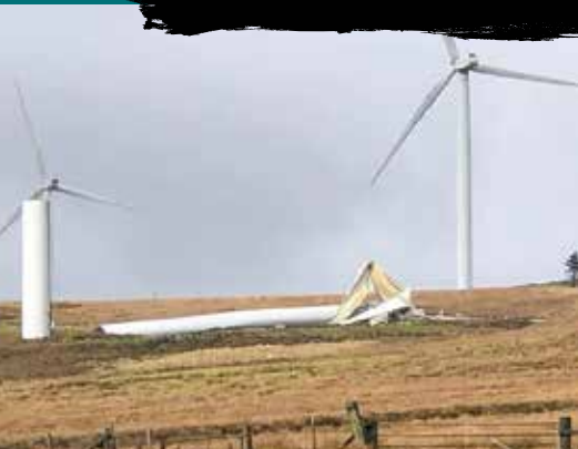
AUSTRALIA TURBINE COLLAPSE
